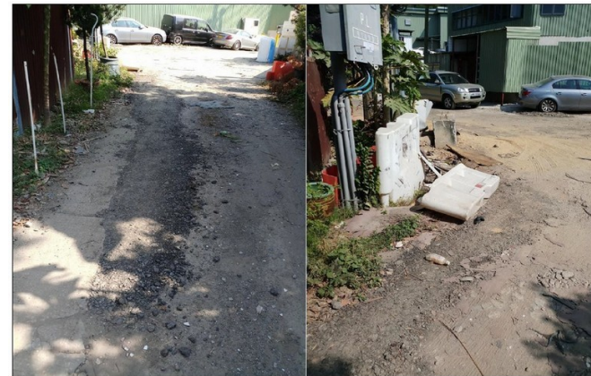
EXISTING SITE CONDITION AT ACCESS ROAD, AFTER COMPLETION OF DRAIN D1
