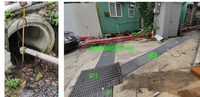
THE STREAM CONNECTS TO UNDERGROUND DRAIN D1A OF 1M DIAMETER
