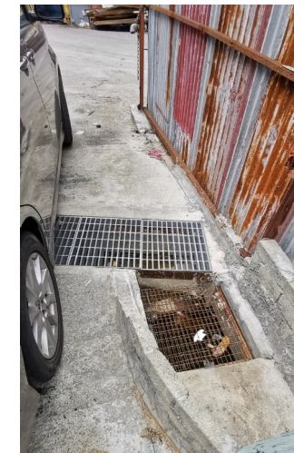
Photo 6 Drain B1 (left), min. 400x400 Drain B4 open channel with grating 400W x 300D Last Manhole ST2 which connects to 600mm pipe D1 shown above
