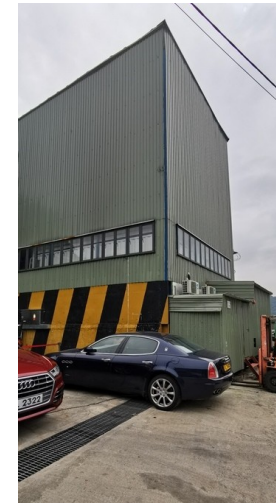
Photo 6 Drain B1 (left), min. 400x400 Drain B4 open channel with grating 400W x 300D Last Manhole ST2 which connects to 600mm pipe D1 shown above
