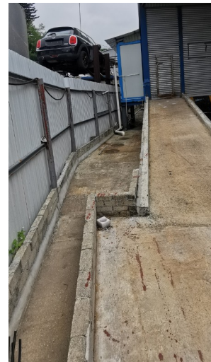
Photo 6 Drain B1 (left), min. 400x400 Drain B4 open channel with grating 400W x 300D Last Manhole ST2 which connects to 600mm pipe D1 shown above
