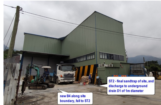
Photo 5 Drain B4 and Last Manhole ST2 during construction
