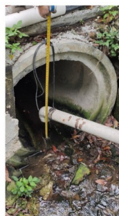
THE STREAM CONNECTS TO UNDERGROUND DRAIN D1A OF 1M DIAMETER
