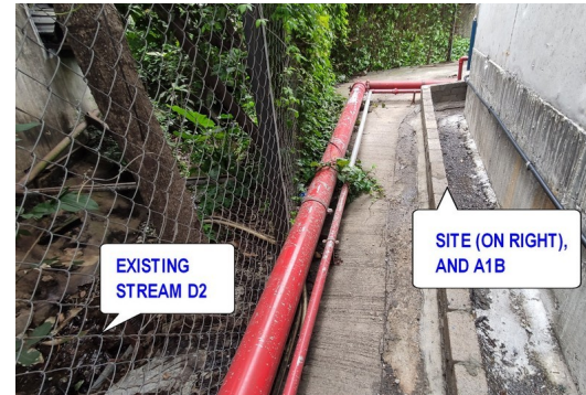
Photo 1 CONDITION OF STREAM D2 (OUTSIDE SITE), AND A1B OF SITE
